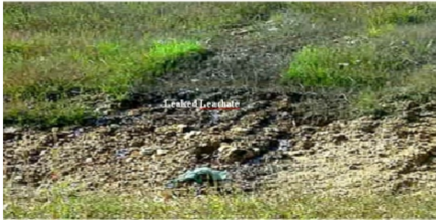
Fig. 1: Seepage of leachate (black) through a weak spot in the landfill cover (Freudenrich, 2010)
