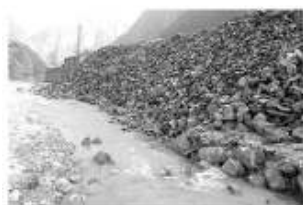
Fig. 1: Spoil heaps lead to the river blockage
