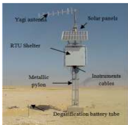
Fig. 8: Onsite RTU equipment
