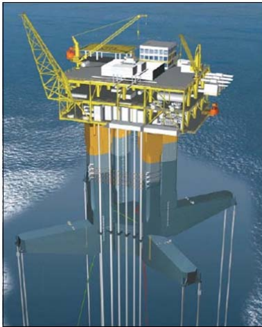
Fig. 6: A typical tension leg platform (Net Resource International Ltd., 2012)
