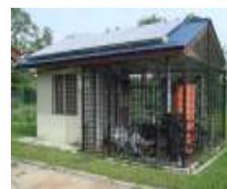
Fig. 25: Photograph of solar dryer using dehumidification system
