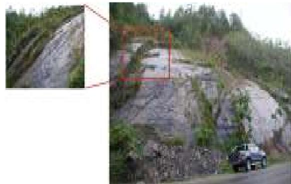
Fig. 4: Rockslide causes by out-dipping of joint planes at station B20
