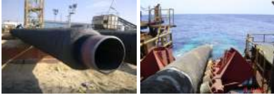
Fig. 1: Concrete Weight Coating (CWC) for offshore pipeline
