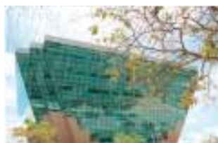
Fig. 3: The energy commission diamond building, Xin and Rao (2013)
