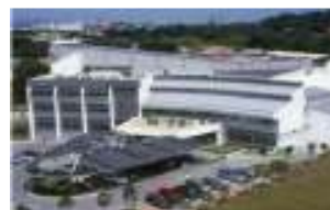
Fig. 1: The PTM (ZEO) building in Bangi, Malaysia, GEO (2011)
