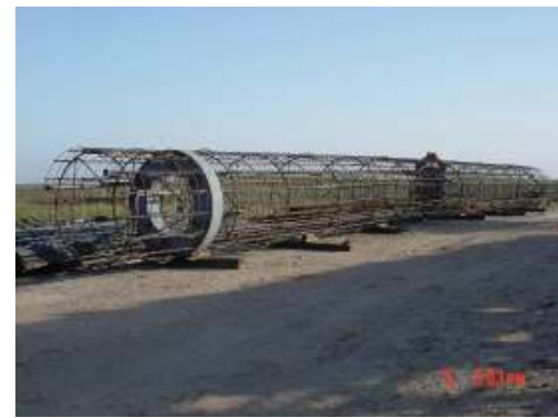
Fig. 3: Welding of load cell in Lanqi bridge
