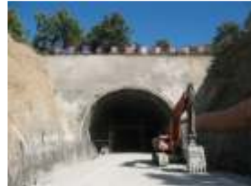
Fig. 5: Entrance of GAOLING Tunnel
