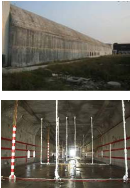
Fig. 1: Exterior and interior view of the test tunnel
