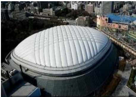
Fig. 2: Japan Tokyo indoor baseball stadium
