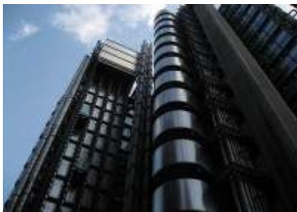
Fig. 3: Lloyd's building in London Richard Rogers Company
