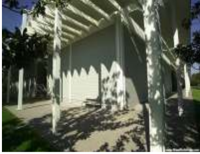
Fig. 1: Concrete light crusher at Menil complex-Renzo Piano
