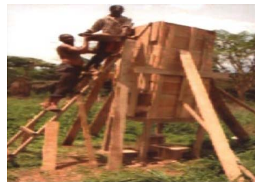
Plate 3: Assembly of box and loading of the frame
