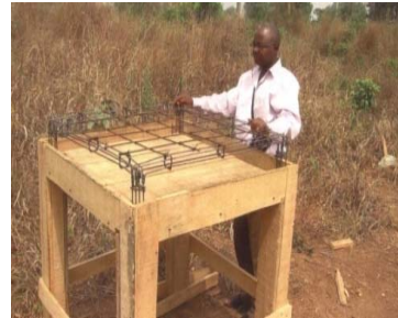
Plate 1: The construction of form work and reinforcement
