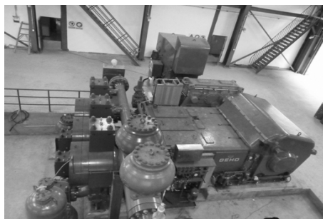
Fig. 1: Diaphragm pump
