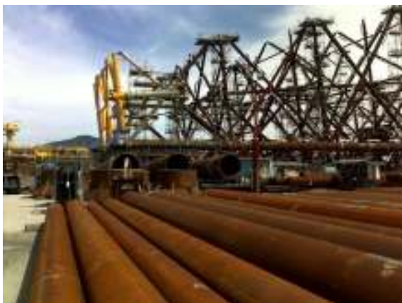
Fig. 2: Data collection for diameter and thickness of tubular members of jacket platform at fabrication yard
