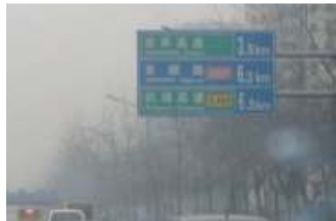
Fig. 1: Inadequate height of English letters in guide signs
