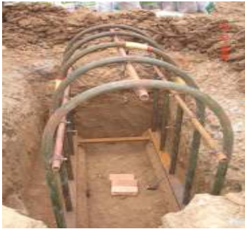
(b) Normal support structure
