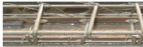
Fig. 1: Local construction of PBH shear connectors
