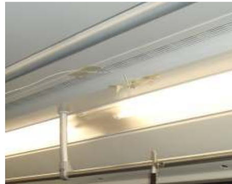
Fig. 5: Vibrate test point collocation at air condition units
