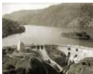
Fig. 4: Water coming from Bhimtal Lake which supplies the water to the water mill
