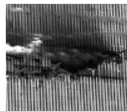
Fig. 1: A ‘clean’ cut driven by the wings of a boeing 767 into the facade of the north tower
