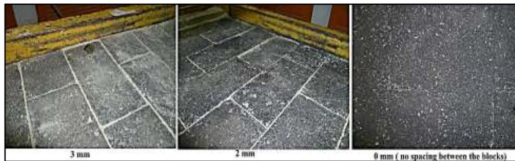
Fig. 2: Asphalt blocks are laid with different joint widths
