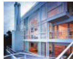
Fig. 9: The Western glazed facade showing the white concrete, glass and stainless steel pipes for the chimney copyright Richard Meier
