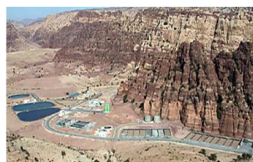
Fig. 2: General view of the Petra Wastewater Treatment Plant location
