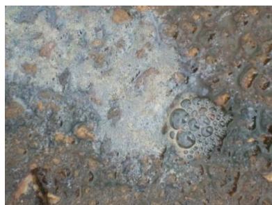
Fig. 7: Methane bubbles from the seeping leachate
