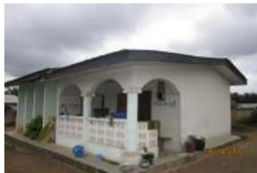
Fig. 5: 5-year old compressed block building at Awunakrom (In this type of structure the earth material is stabilised by compaction to increase density and strength)
