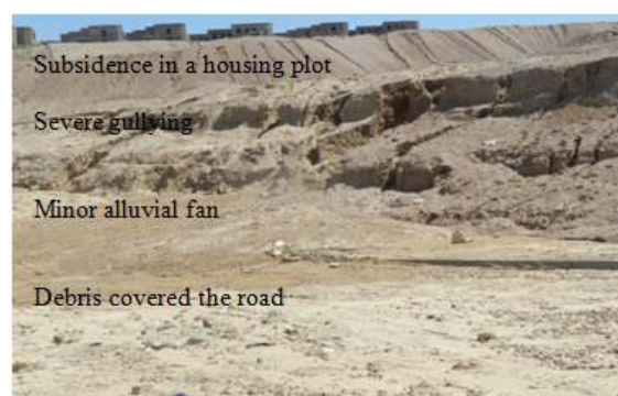
Fig. 12: Minor alluvial fan, severe gullying, road covered with debris and subsidence of a housing plot
