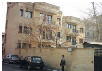
Fig. 3: A typical and modern building with shared courtyard (Mirmoghtadaee, 2009)
